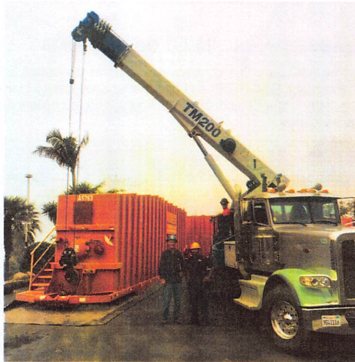
Figure 3: Parking area tankage
