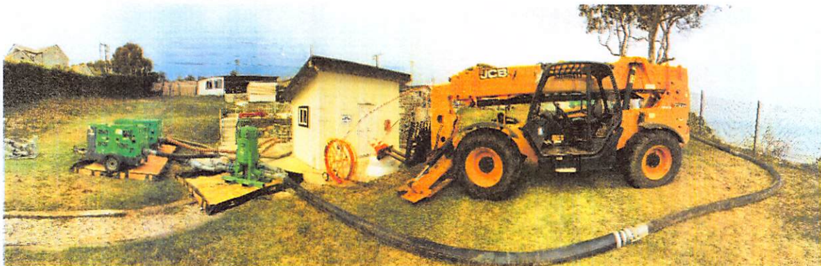
Figure 4: Panoramic of Lower Equipment Spread
