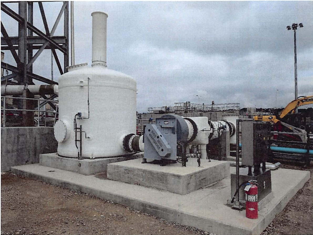
Figure 5.21 DCWater Carbon Adsorber Odor Control System
