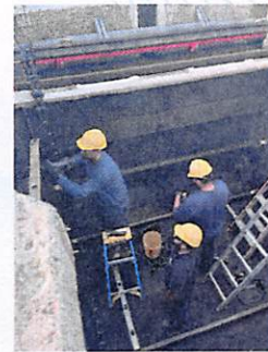
New Sprockets for Primary Clarifier
